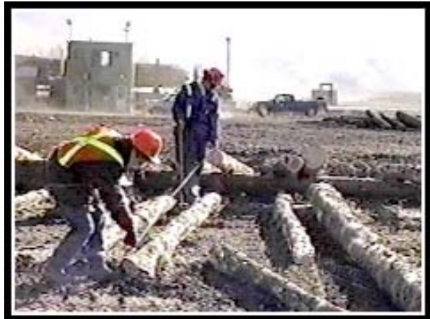
Logs laying flat on ground increases back bending and increases risk of injury.
